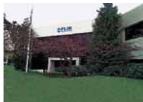
FLIR Systems, Portland
